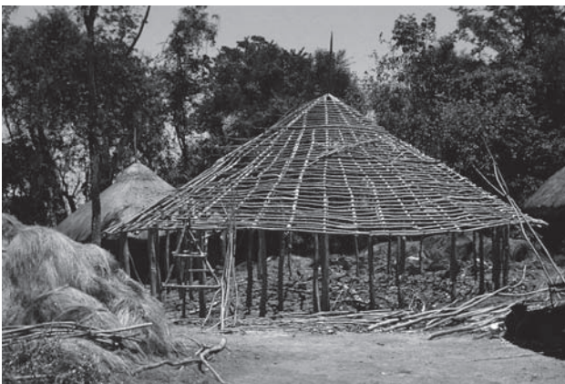
Figure 4. A Luo house ( ot ) under construction, with materials gathered for the project.
